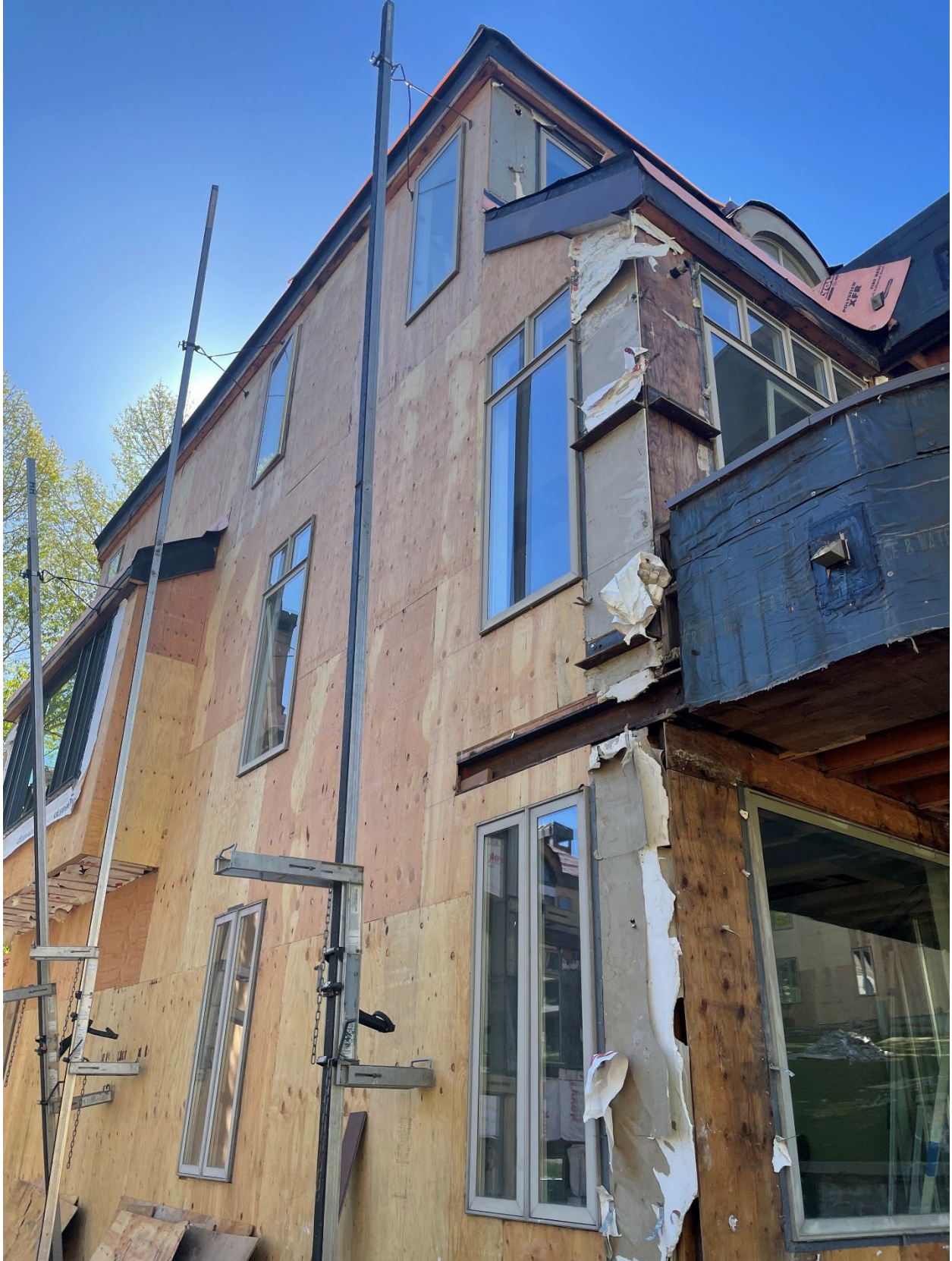
Northwest corner Unit B5
